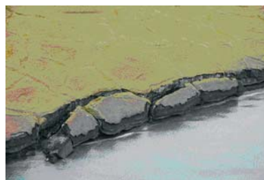
FIGURE 1. Block failures such as this one to the west of Komakuk Beach are common along the Yukon Coast. These failures usually occur along ice wedges (indicated by the troughs on the tundra surface) and the exposed ice wedge can be seen near the top of the coastal bluff. Now that the block has fallen to the beach, it is more easily eroded by waves, and the sediment and soil carbon will be washed into the ocean.
