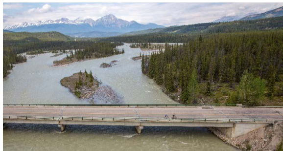
Cyclists on the existing Icefields Parkway.
