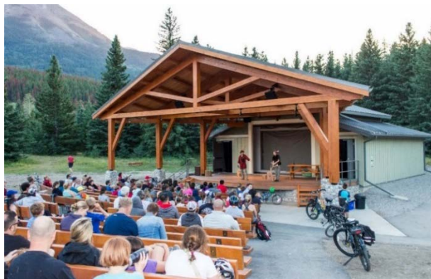
The new amphitheatre at Whistlers Campground was completed in July 2017.
