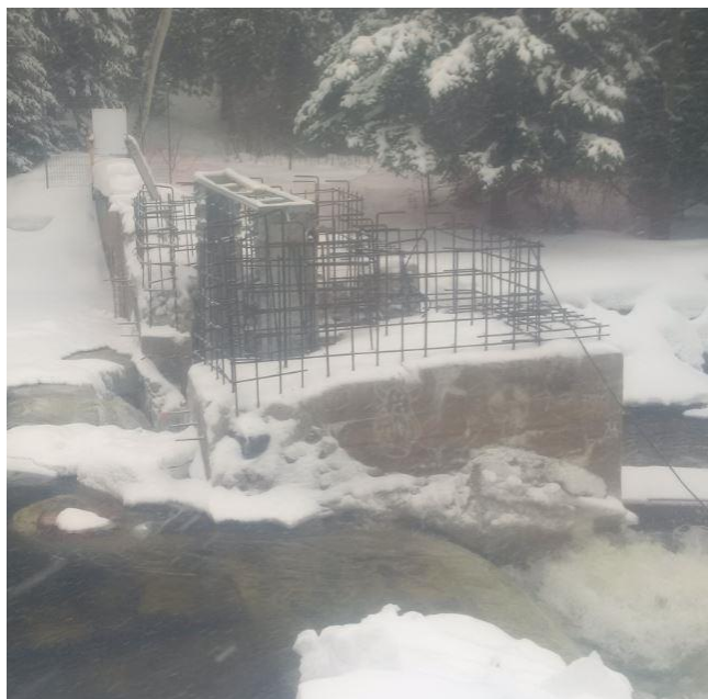
New Dam's Formwork
