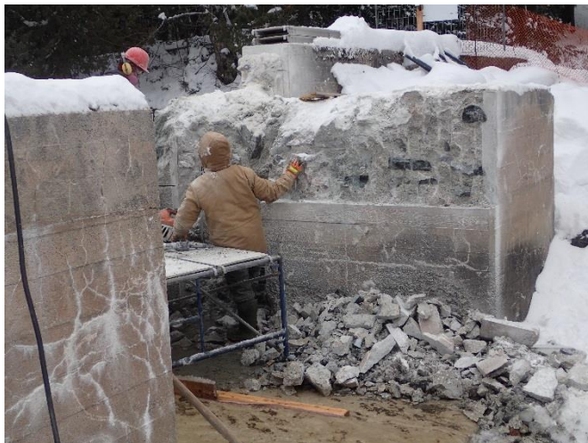
Removing Damaged Concrete
